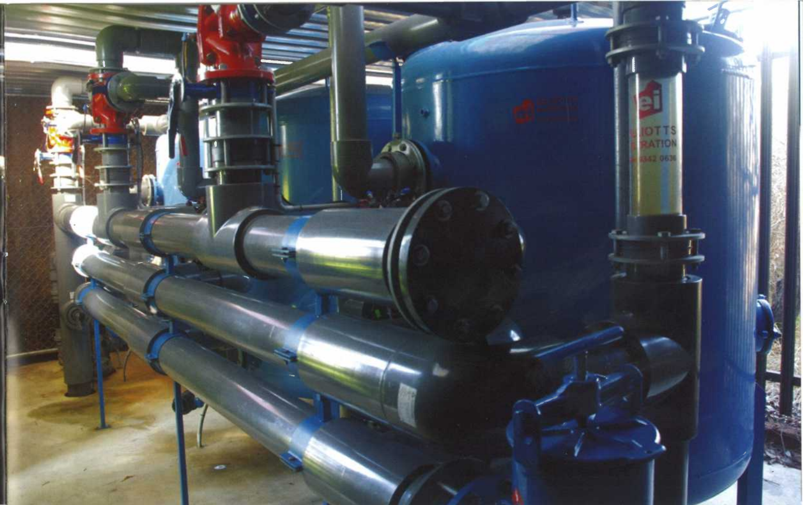
Above: Commissioning of the iron filter at Vasto Reserve, Stirling - WA
